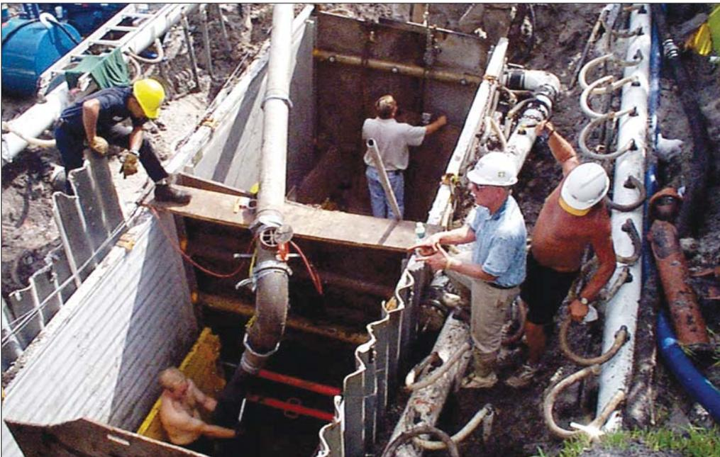
Moreover, the so-called "conventional" open-cut method sometimes takes less conventional forms, based on the specific demands and constraints of a job. For example, for an emergency repair to a collapsed sewer main in Pembroke Pines, FL, the hydraulic excavator capable of performing such a deep repair could not access a rear-yard easement due to close spacing between residences. Instead, high-powered vacuum excavation equipment was utilized, as shown in the photo to the left. ▀
