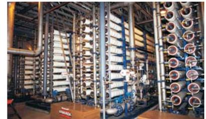
Above: Reverse Osmosis High-Pressure Pumps and Ion-Exchange Vessels.
