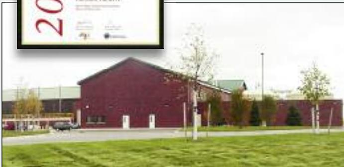
In service since July 2005, this facility improves water quality in the Detroit River by ending the discharge of untreated overflows into Conner Creek, a tributary of the river. The facility has 30 million gallons of storage capacity and includes screening, disinfection, settling, skimming, flushing, and dewatering systems. Existing outfalls were rehabilitated and reused, which added another 32 million gallons upstream of the facility.
