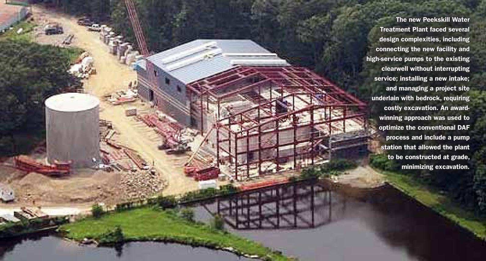
The new Peekskill Water Treatment Plant faced several design complexities, including connecting the new facility and high-service pumps to the existing clearwell without interrupting service; installing a new intake; and managing a project site underlain with bedrock, requiring costly excavation. An award-winning approach was used to optimize the conventional DAF process and include a pump station that allowed the plant to be constructed at grade, minimizing excavation.
