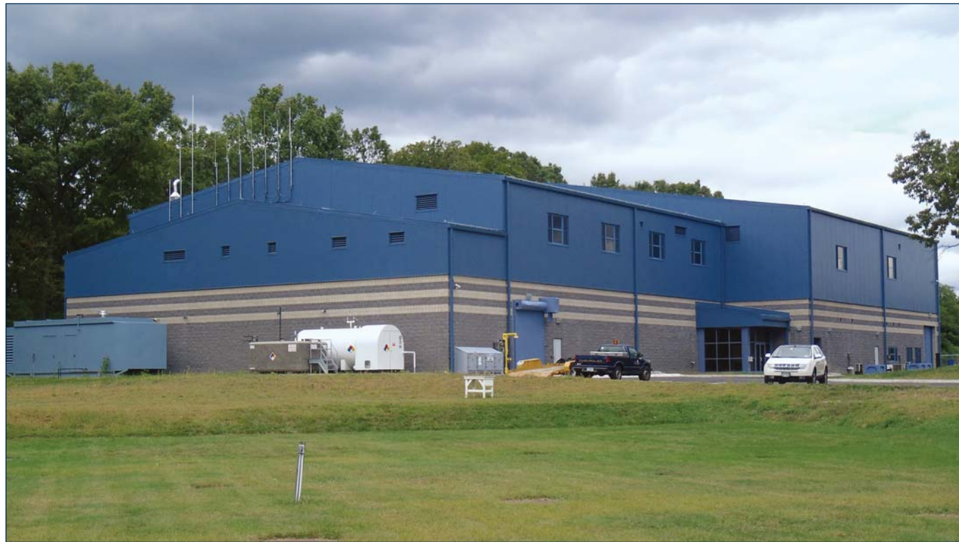
The new Peekskill Water Treatment Plant began serving customers in May 2010, utilizing a cost-effective treatment process that efficiently removes organics and produces a finished water that consistently meets Disinfection By-Product limits that had been seasonally exceeded by the old plant.
