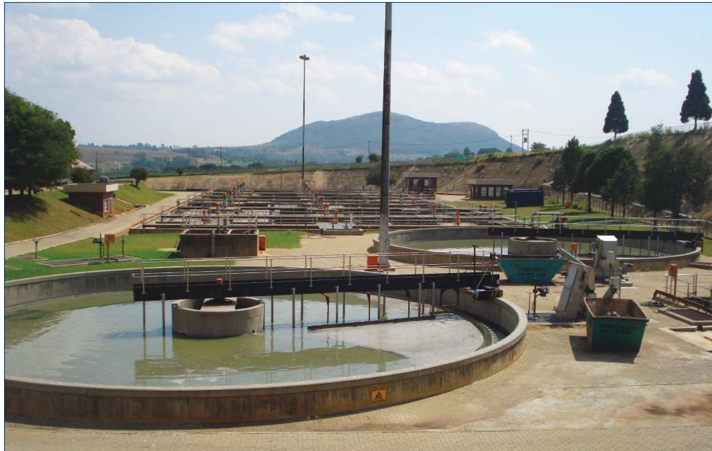
The Driefontein Wastewater Treatment Plant, which was honored in 2004 as South Africa's best-operated treatment facility, is undergoing upgrades and expansion to 55 MI/d (from 35 MI/d).
