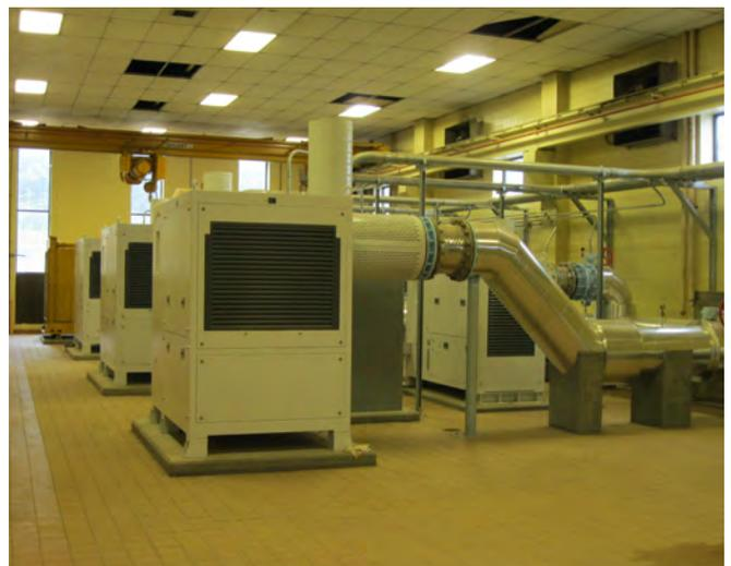
**Existing engine-driven blowers were replaced with high-speed direct-drive centrifugal blowers driven by electric motors.** Hazen and Sawyer
