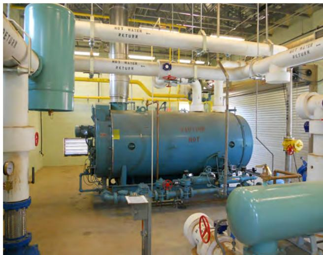
**One hot-water boiler was provided to supplement digester heating during cold weather. During winter, biogas from anaerobic digestion is used to fire the boiler.** Hazen and Sawyer
